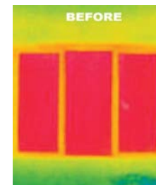
Heat is being lost through inefficient windows and doors
